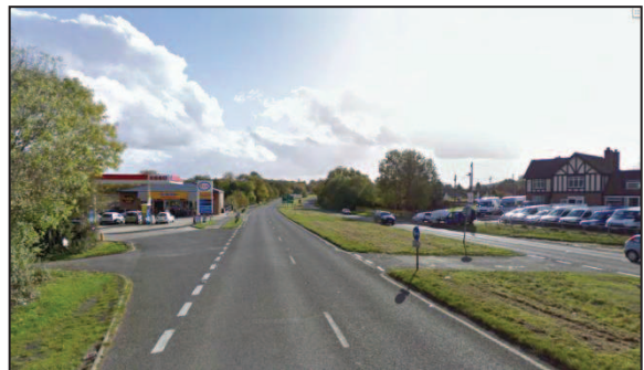
Photo 2 – safety issues by petrol station A24 view southbound
